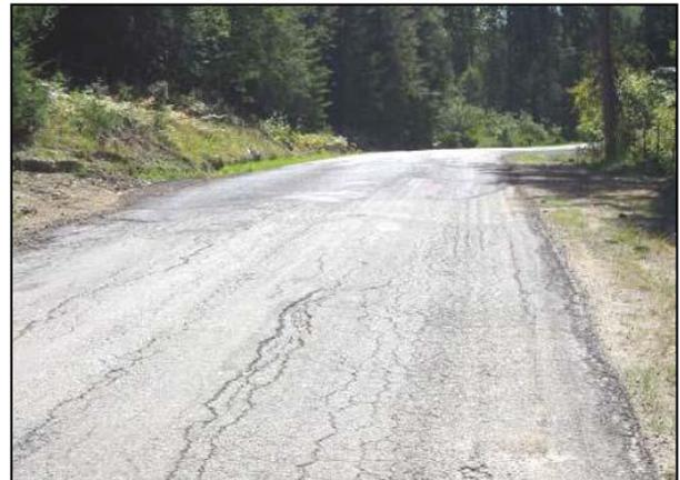
Figure 2. Example of pavement with base problems. (Photo courtesy of the Portland Cement Association (PCA)).
